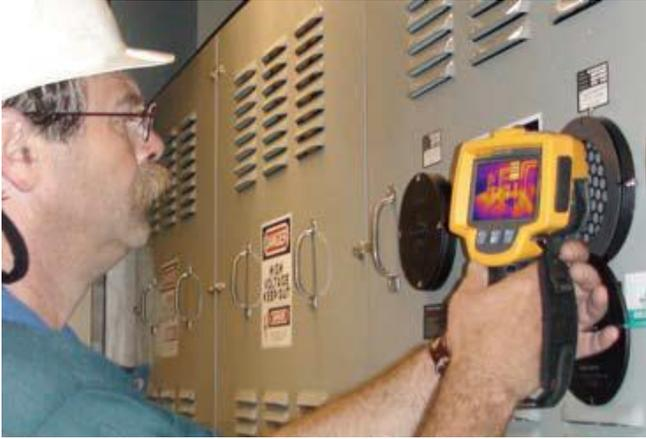
**Example of a thermographer using an IR window and wearing standard level of PPE required while operating energized electrical equipment in an enclosed and guarded condition.**
